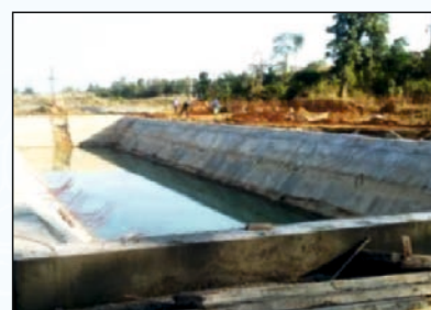
Permanent Settling Tank
