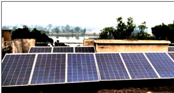
9 Kwp solar panel installed at Roof-top
