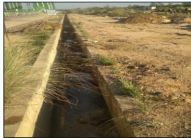
Concrete Drain
